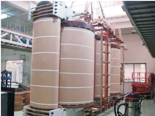
• Transformer body after assembly
