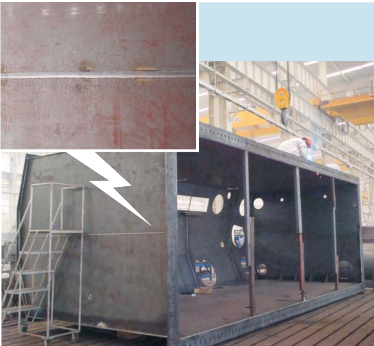
• 220kV Bell type oil tank under welding
