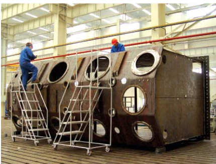
• Welding of 220kV oil tank
